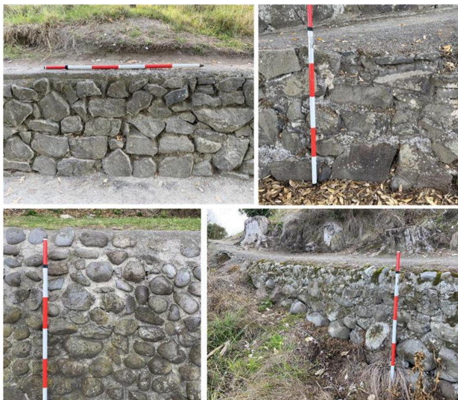
Figure 4 – Comparison of wall masonry styles. Clockwise from top left: Wall 1, Wall 5, Wall 8 and Wall 11.
