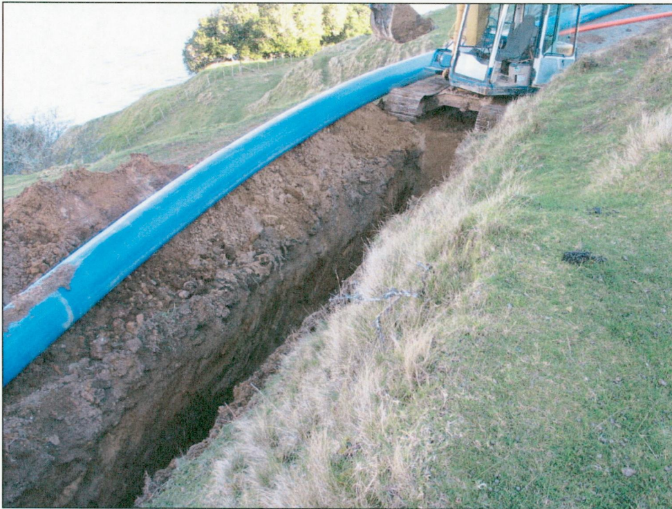
Figure 7. Water main installation 2010. (K. Phillips 2010)
