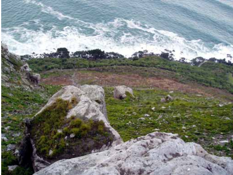
Photograph No 22; Unstable column at 3d.
