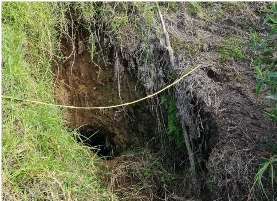
Photo 2; The sinkhole at the surface (2m scale).
