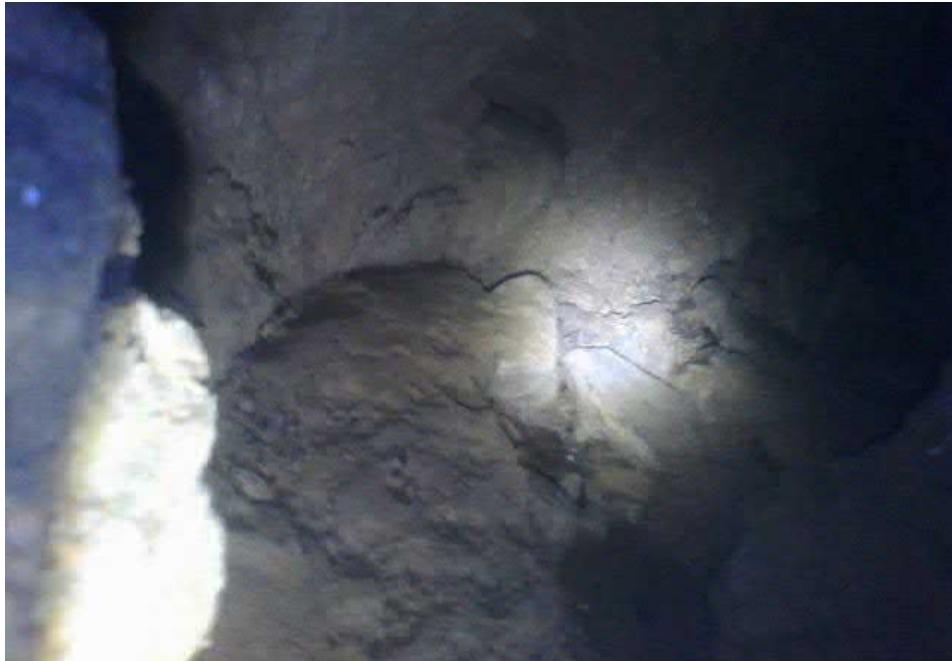
Photo 5; The tunnel continues to the right. Furthest view in photo is around 5m from the entrance. The diameter of the tunnel here is around 0.5m.
