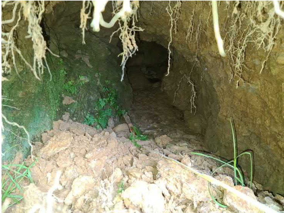
Photo 3; The sinkhole entrance.
