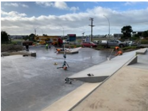
Gordon Spratt Skatepark Under Construction constructors
