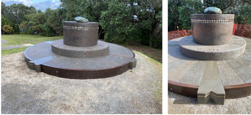
Celestial Compass installation was completed on the summit of Mauao, in time for Matariki.
