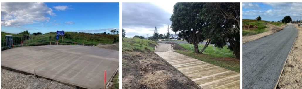
Construction progress on the Papamoa Shared Path.
