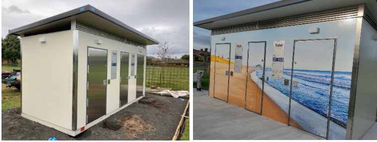
New toilet block installed, and with wrap applied
