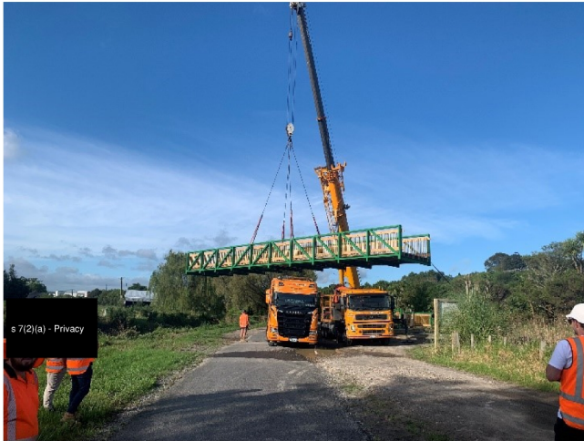
New Pedestrian Bridges arriving at site and ready for installation
