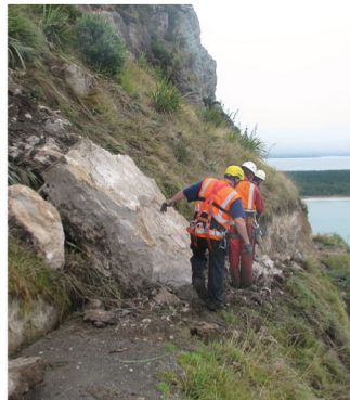
Staff chased down the loose rock remains to ensure the safety of people using the track below.
