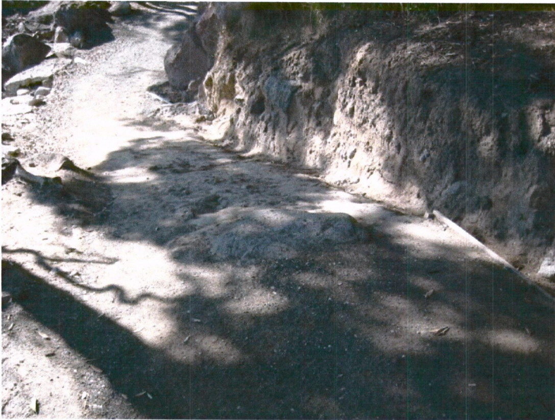
Foot traffic wear of the track surface, especially on steep sections Provision of an asphalt surface is the best long term low maintenance option
