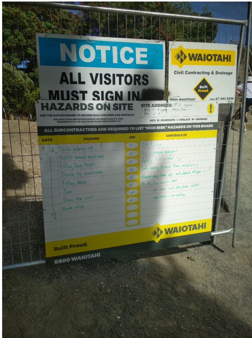
Figure 8:9: Front Facing and Hazard Board
