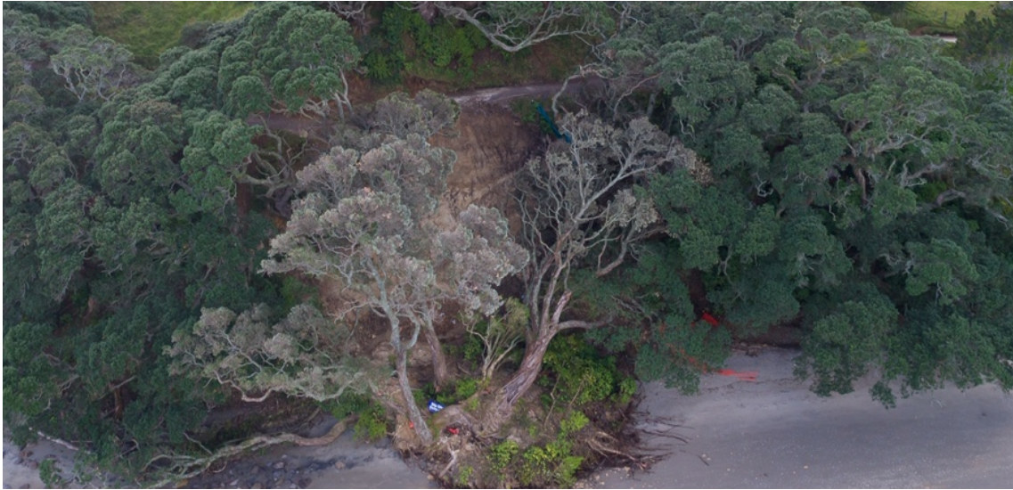
Figure 8:1: Mauao Slip, Prior to Physical Works (Tauranga City Council)
