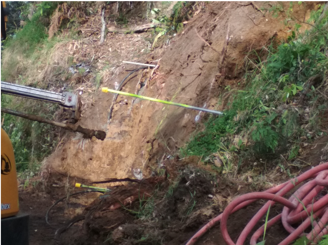
Figure 8:12: Drilling and Inserting Soil Nails
