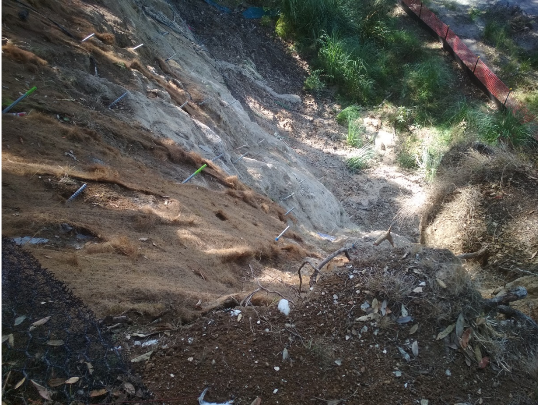
Figure 9:1: Soil Nails in Lower Bank
