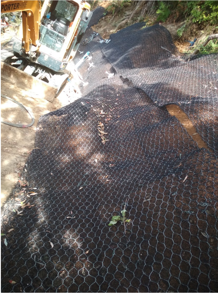
Figure 8:13: Mesh, Backing Plates
