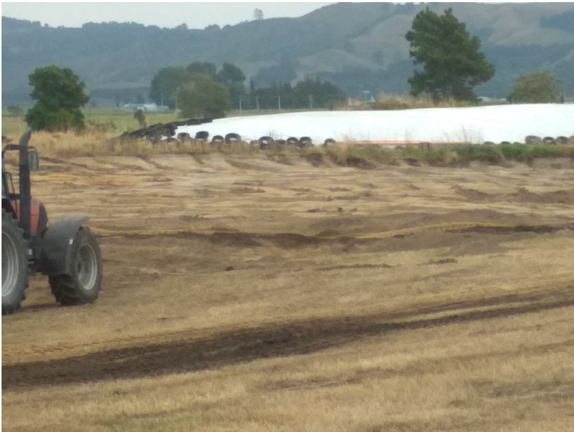
Figure 9:3: Pond G at Start of Works
