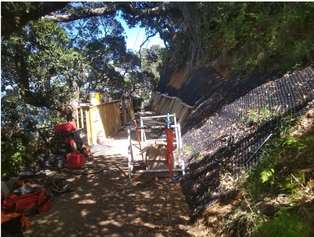
Figure 9:2: Track and Upper Slope
