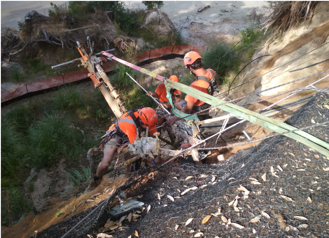
Figure 8:20: Soil Nail Drilling and Abseiling
