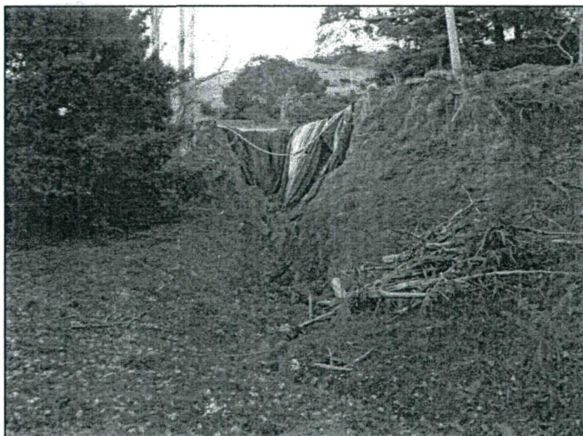
Figure 8. View of Slip 2 looking up to the black polythene covered erosion scarp on the 4WD track.
