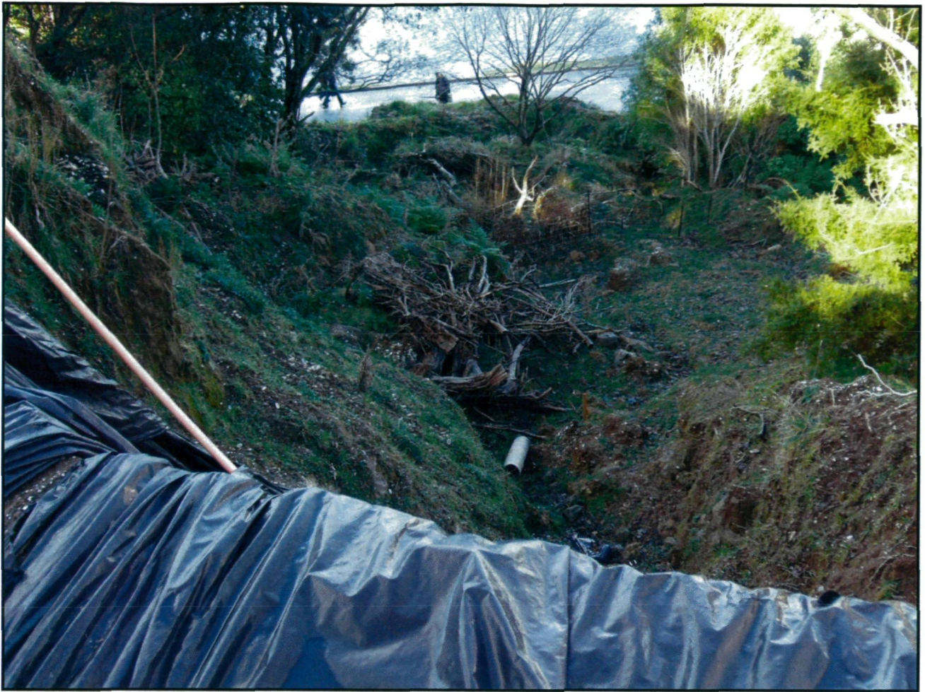
Figure 6 Looking down the slip
