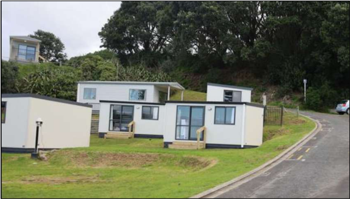
Figure 4: Example Photo of 15.4m 2 basic MAUs without decks on existing camp sites 113, 114, 123 and 124 (Source: section 2.3 on page 13 of AEE)
