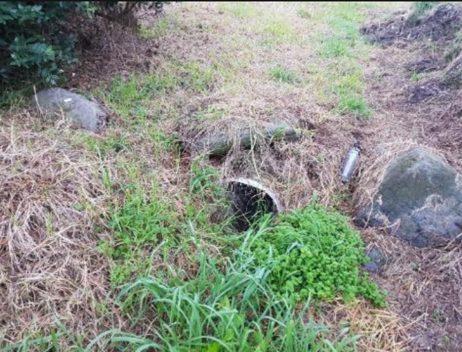
Current Storm-water Inlet
