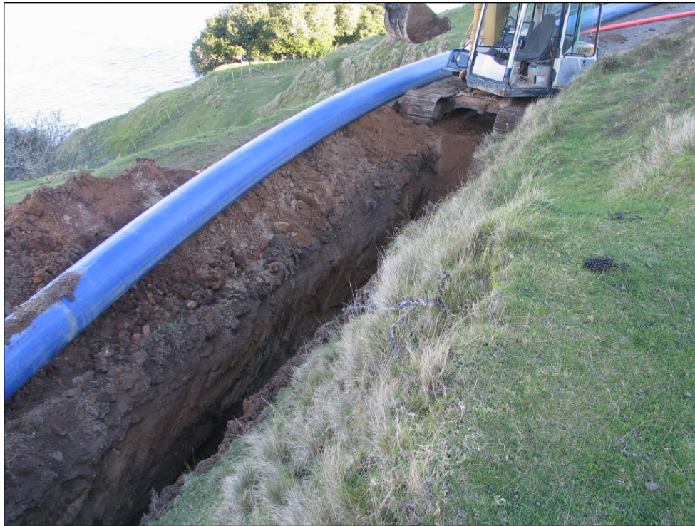
Figure 7. Water main installation 2010. (K. Phillips 2010)
