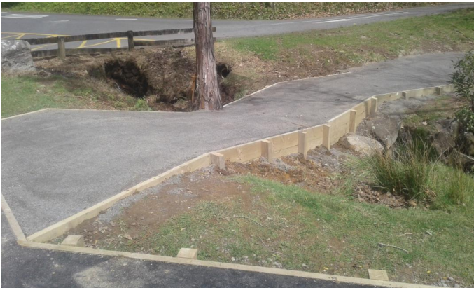
Realigned track alleviating the need to maintain a structure
