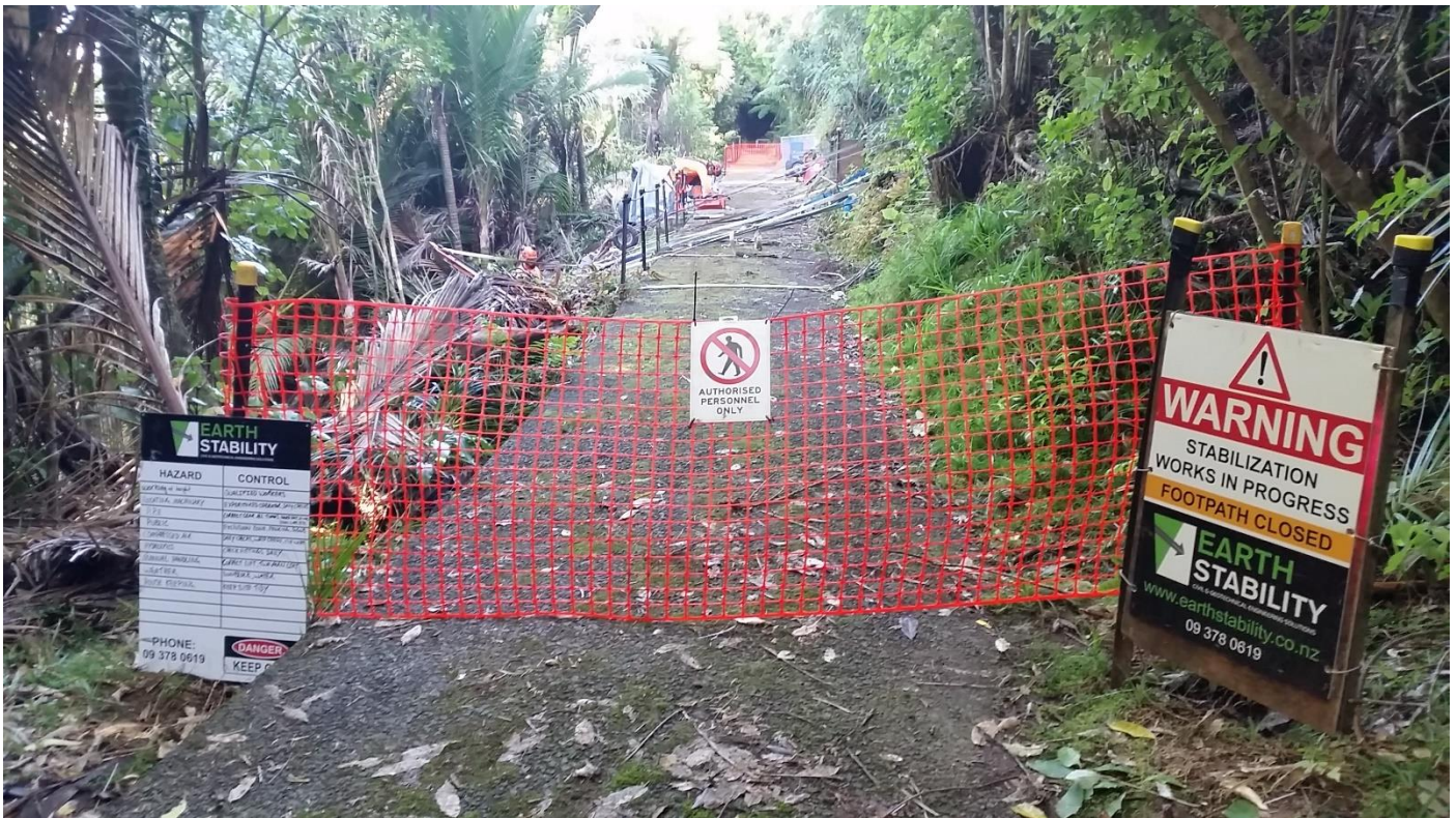
Figure 1 – Site safety signage at track closure point.
