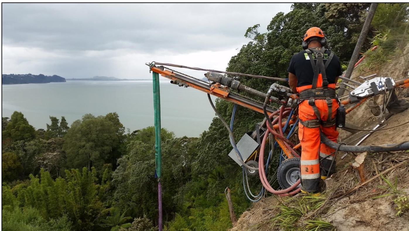
Figure 2 – Restricted access drill rig
