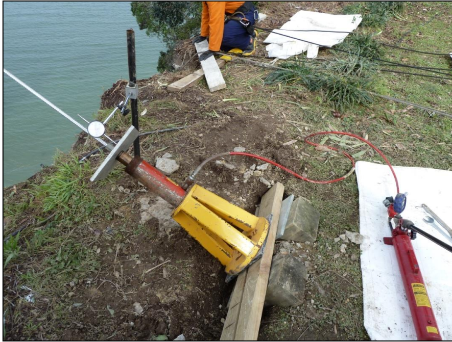
Figure 3 – Testing of soilnails
