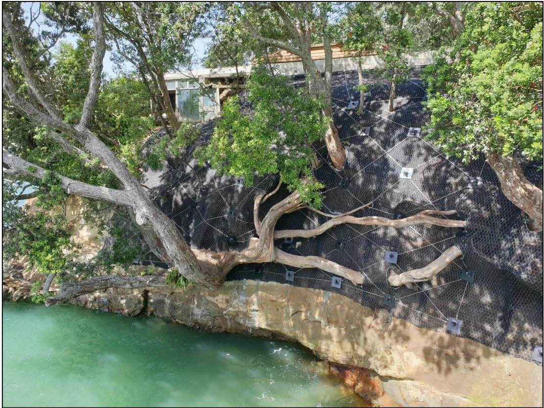
Figure 5 - Example of Duramat RF Installed in a coastal environment
