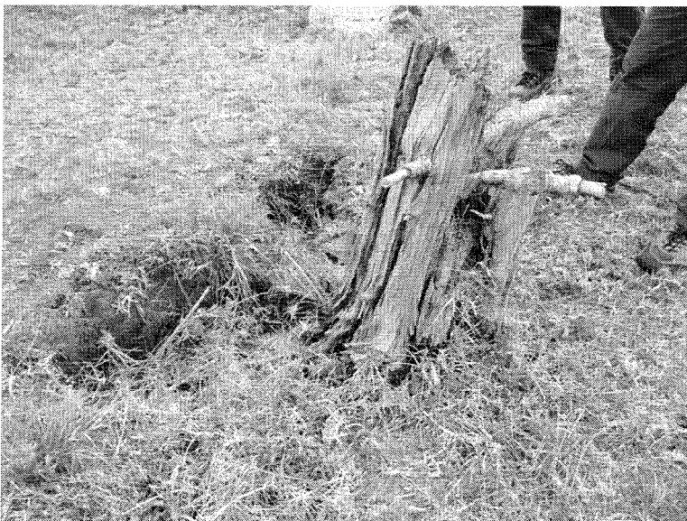
Photograph 3. Localised subsidence due to decaying root systems.
