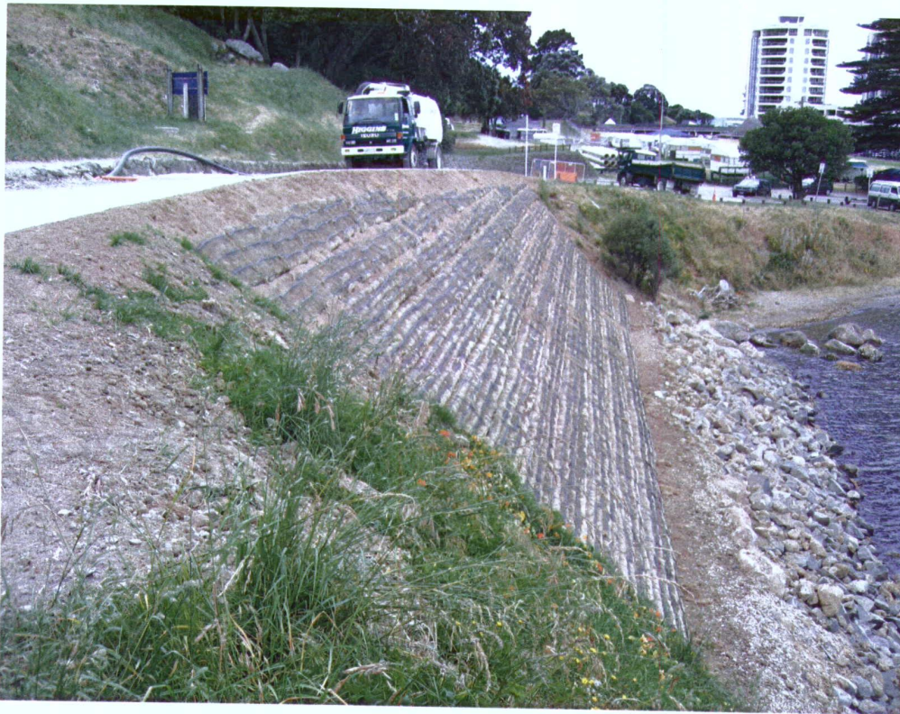
Photograph 2; Repair completed to dropout wharf access road.
