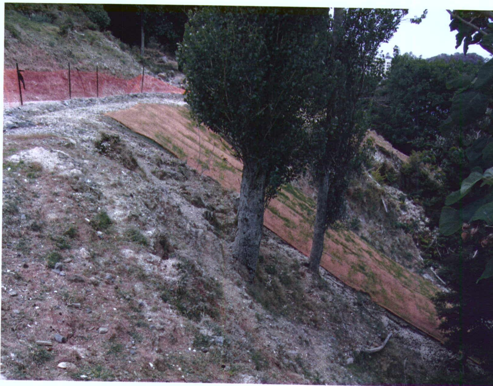
Photograph 1; Repair completed to dropout on lower 4WD track.
