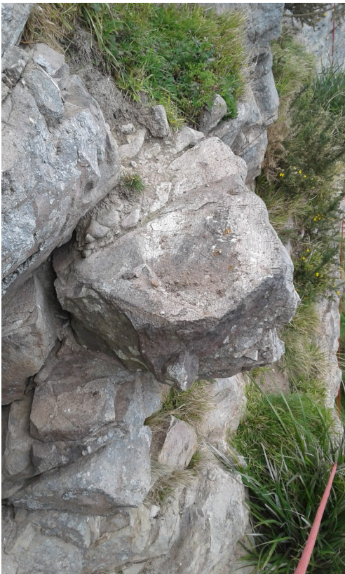
Photo 2. Loose rock previously identified above the Oruahine track.
