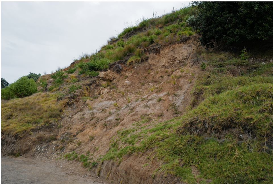
Photo 3. Recent erosion control planting.
