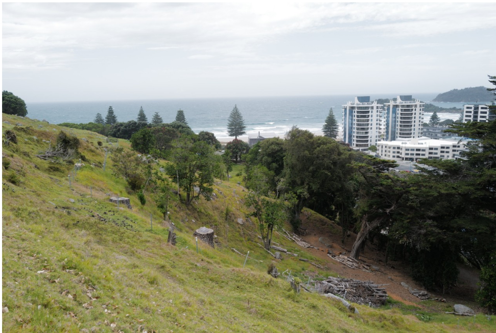
Photo 1. Tree felling completed.
