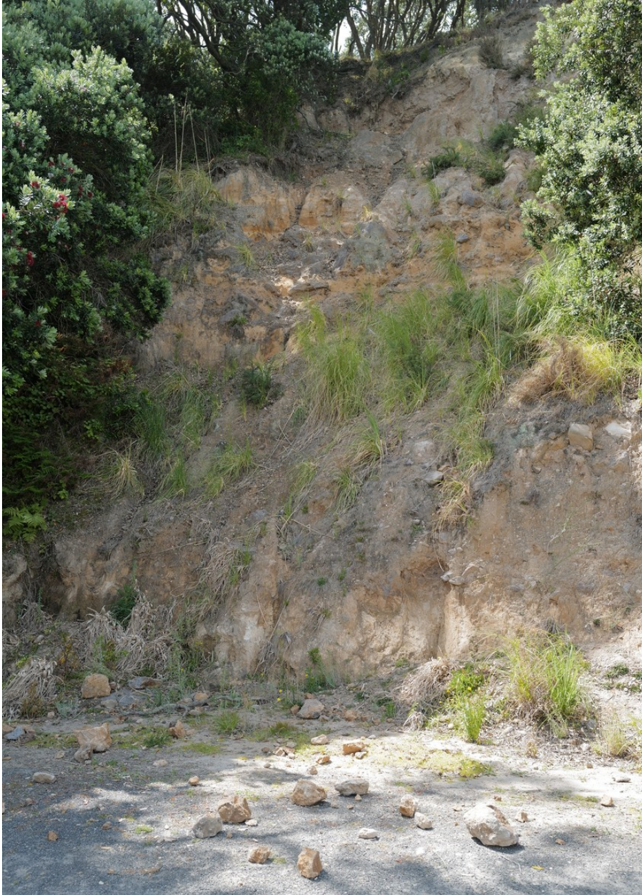
Photo 4. Scaling and weed spraying was completed on 3 December 2019.
