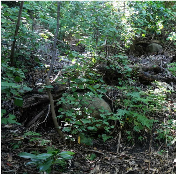
Photo 7. Boulders on the slope surface above the southern base track
