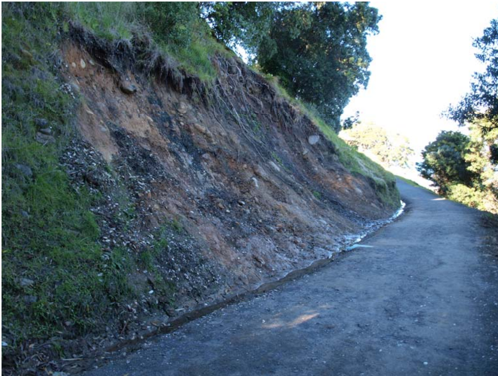
Photograph 8; Slip scars are also still present in places above the base track.
