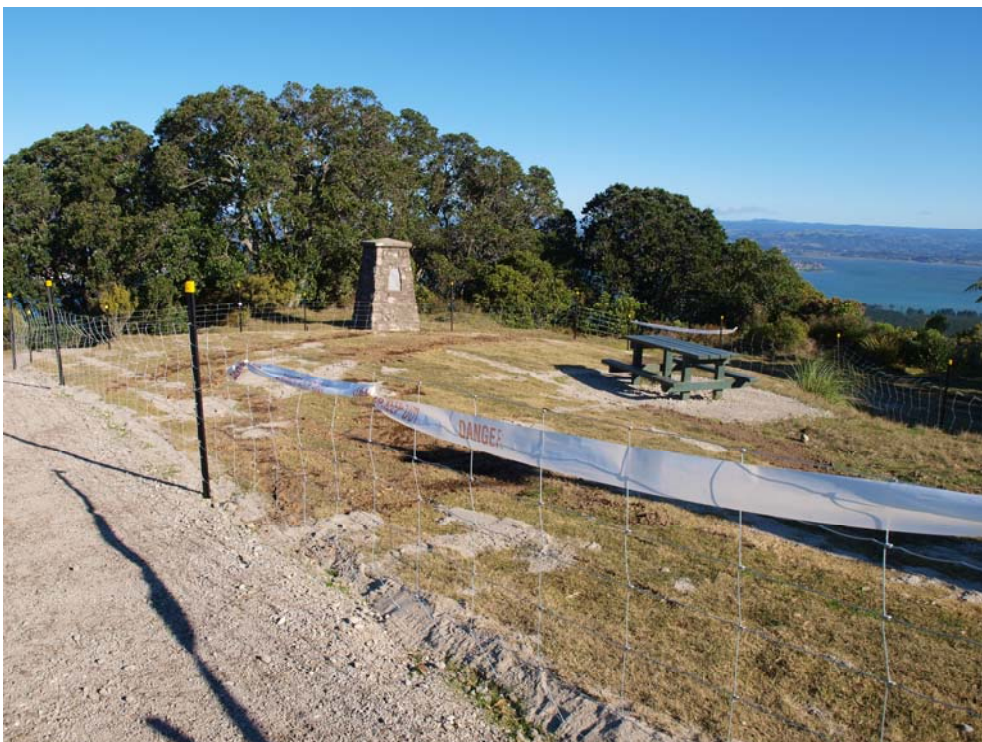
Photograph 11; Erosion control work on summit.
