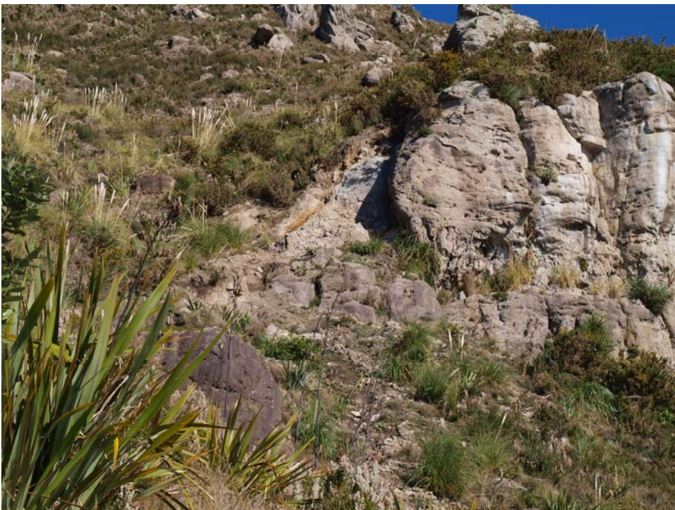
Photograph 5; The site of last years blast scaling; acceptably stable.
