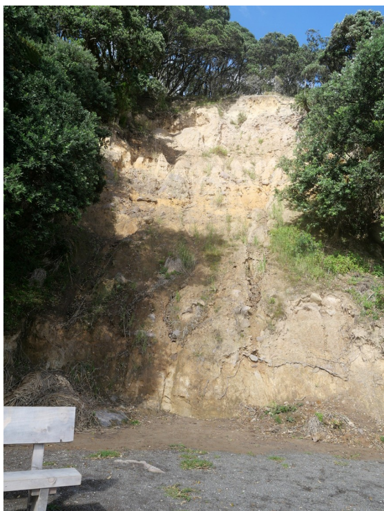
Photo 12. New bench seat below base track slip.
