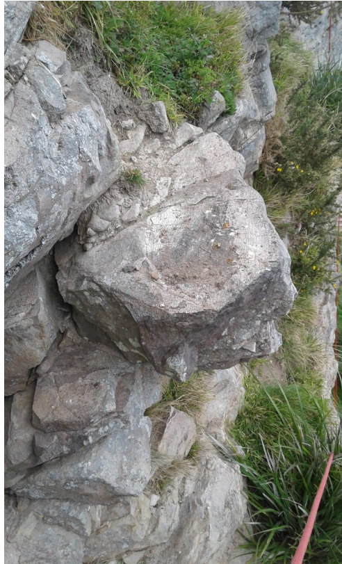
Photo 2. Loose rock above the Oruahine
