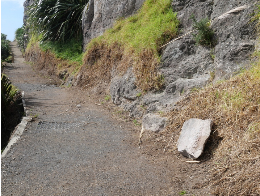
Photo 8. Rock found on Oruahine track.
