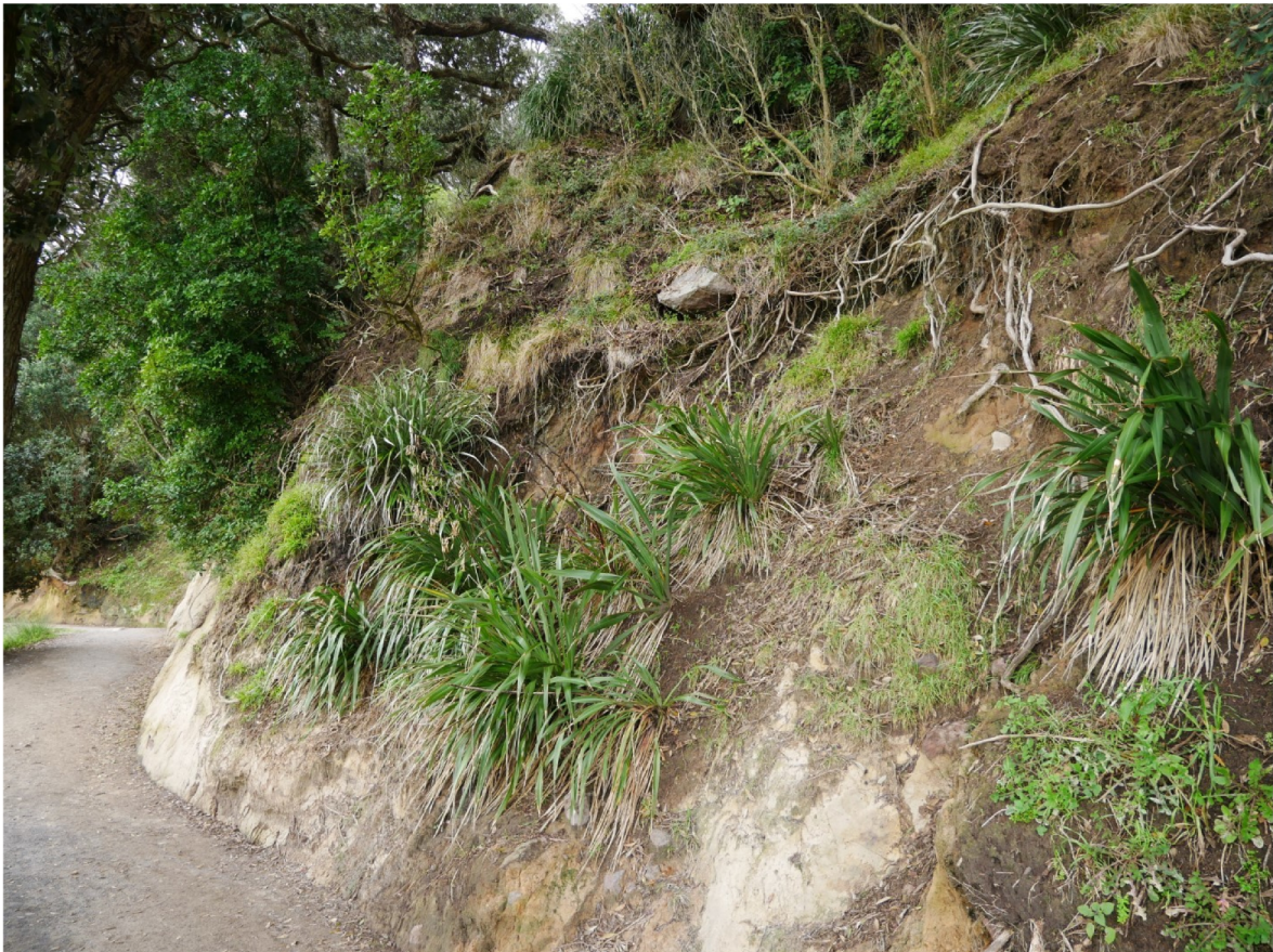
Photo 6; Small rock above base track
