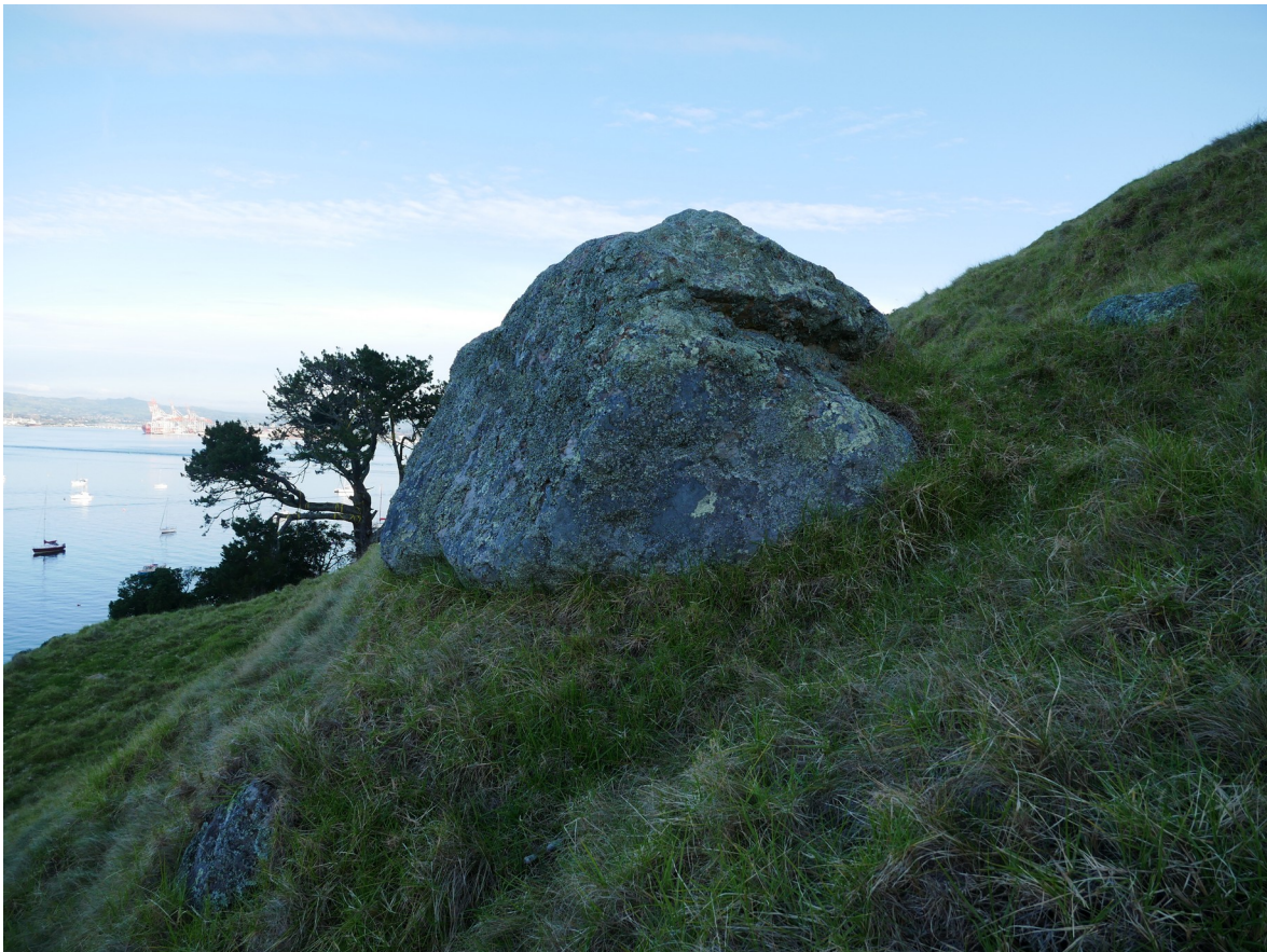
Photo 2; The boulder appears stable at present and has not moved recently.
