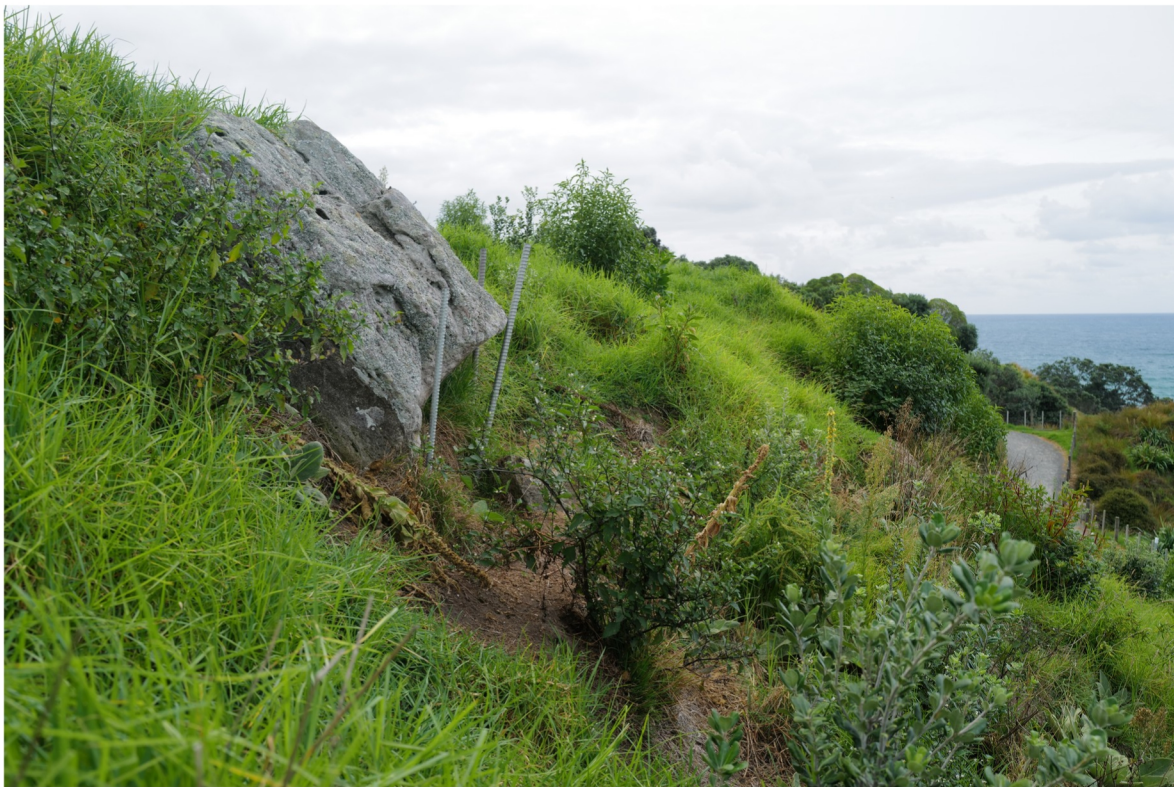
Photo 9; 3m long 25mm diameter pins driven in front of boulder.
