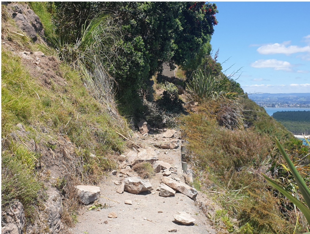
Photo 13; Some of the rock in Photo #12 stopped on the Oruahine track.
