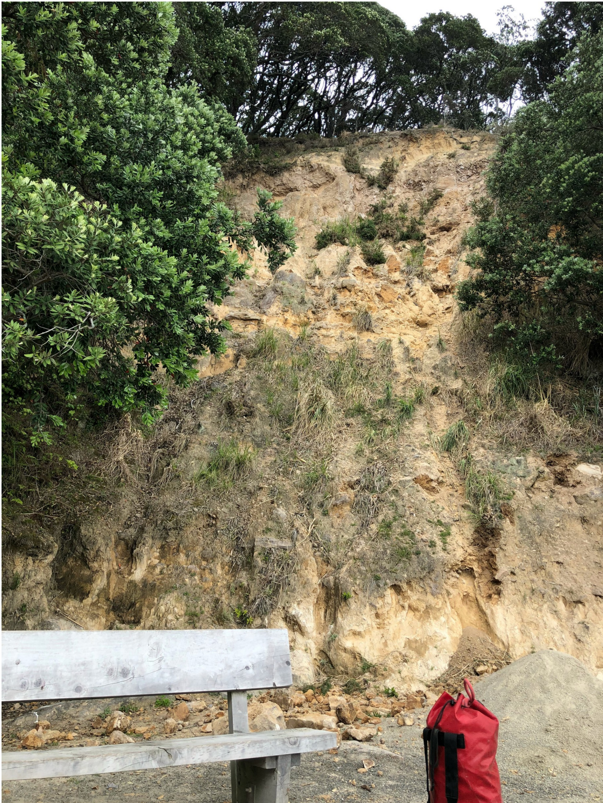
Photo 15; Scoured slope face above the Western Base Track. Fresh rocks are regularly exposed on this slope as the natural weathering process proceeds.
