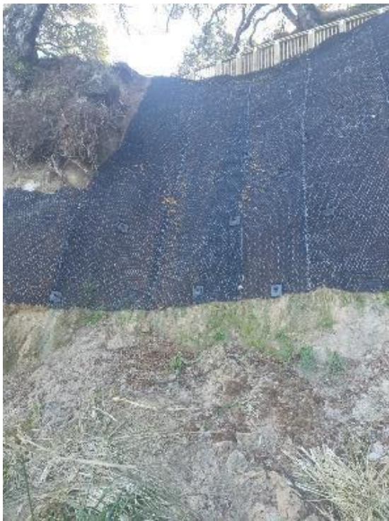
Photograph 7 (top left, taken on 27/08/20) and Photograph 8 (top right, taken on 14/01/21) showing the minor amount of scouring that occurred below horizontal drain 3 during the month of September. Photograph 9 (bottom left) and Photograph 10 (bottom right) show that scour has gradually occurred since the beginning of monitoring to the present.
