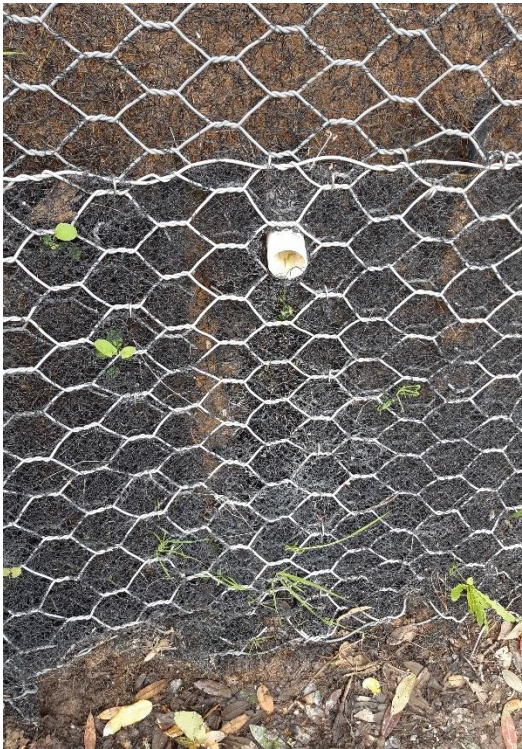
Photograph 10 (top left): Horizontal drain 01. Photograph 11 (top right): Horizontal drain 02. Photograph 12 (bottom left): horizontal drain 03. Photograph 13 (bottom right): looking towards the west end of the repaired track from horizontal drain 01. All photos were taken on 28/09/20.
