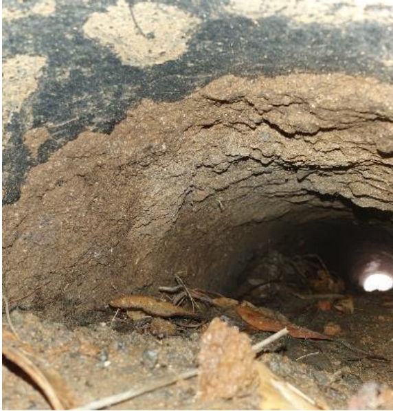
A comparison of Culvert 2 as initially inspected on 02/06/20 (Photograph 11 - above, left) and on 02/08/20 (Photograph 12 - above right). Buildup of material has nearly blocked the drain at the track end.
