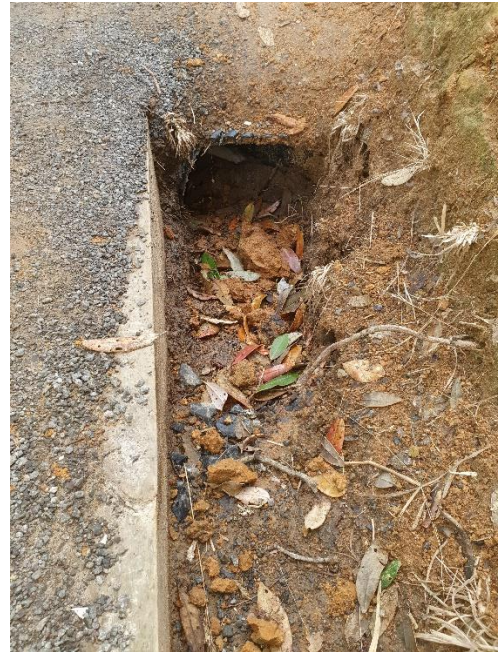
A comparison of Culvert 2 as initially inspected on 02/06/20 (Photograph 9 - above, left) and on 02/08/20 (Photograph 10 - above right). Material from the slope above the drain has been collecting in the slope side of the drain.
