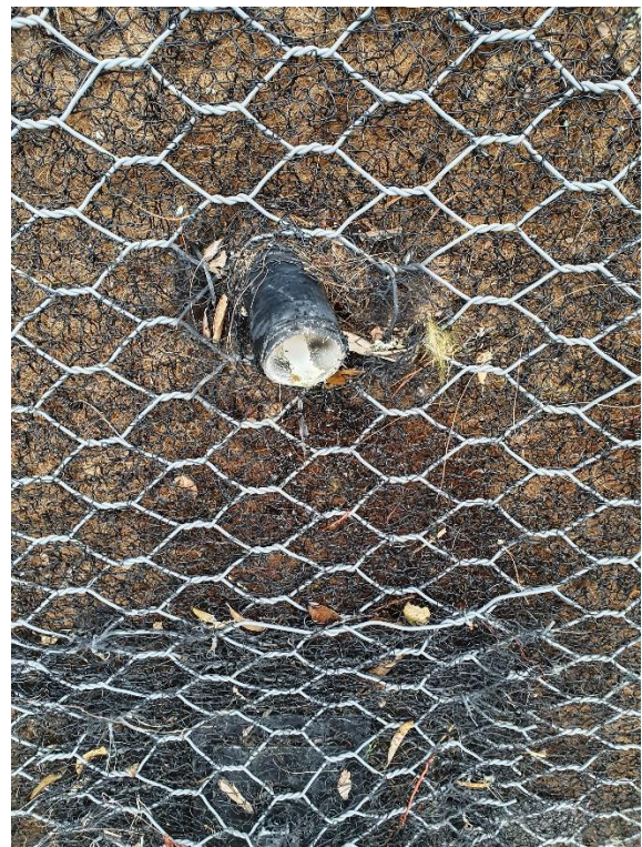
Photograph 5 (left): Water steadily flowing from horizontal drain 01 (HD01). Photograph 6 (right) horizontal drain 02 (HD02) dripping steadily.
