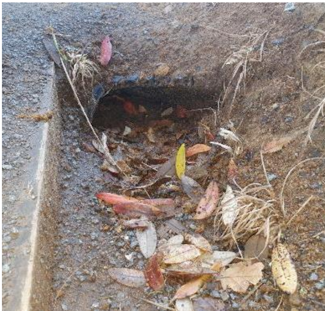
A comparison of Culvert 2 as initially inspected on 02/06/20 (Photograph 9 - above, left) and on 02/08/20 (Photograph 10 - above right). Material from the slope above the drain has been collecting in the slope side of the drain.
