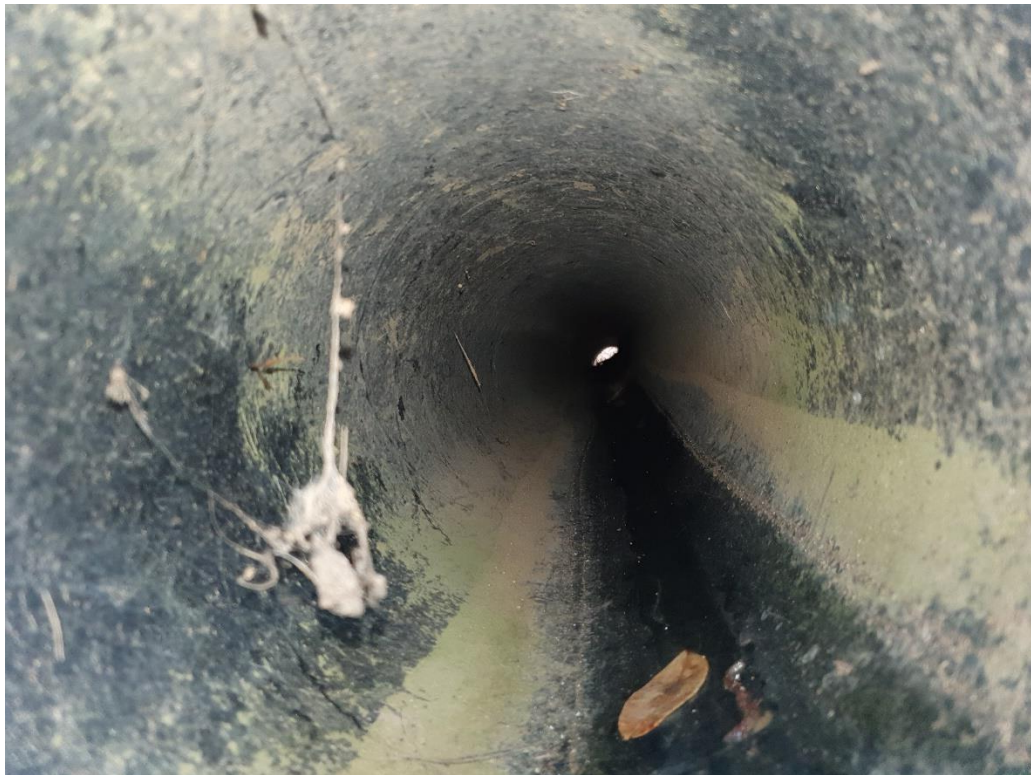
Photograph 13 - culvert O2 looking from the slip side of the track to the slope side of the track. The material has only accumulated at the slope side of the culvert.
