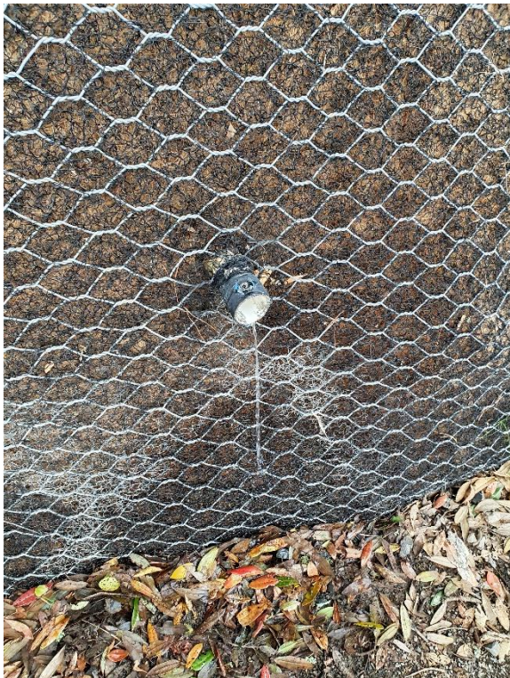
Photograph 5 (left): Water steadily flowing from horizontal drain 01 (HD01). Photograph 6 (right) horizontal drain 02 (HD02) dripping steadily.
