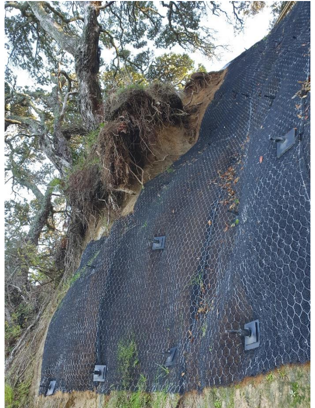
Photograph 10 (left, 02/06/20) and Photograph 11 (right, 29/06/20). Looking west across slip face towards the Pohutukawa tree. It appears that slightly more scour adjacent the tree has occurred following heavy rain.
