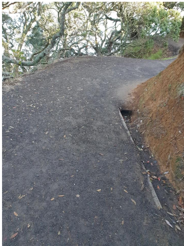
Photograph 3 - Culvert 02 at west extent of track repair
