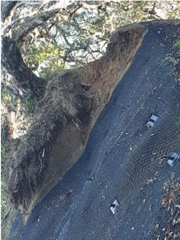
Photograph 10 (left, 02/06/20) and Photograph 11 (right, 29/06/20). Looking west across slip face towards the Pohutukawa tree. It appears that slightly more scour adjacent the tree has occurred following heavy rain.
