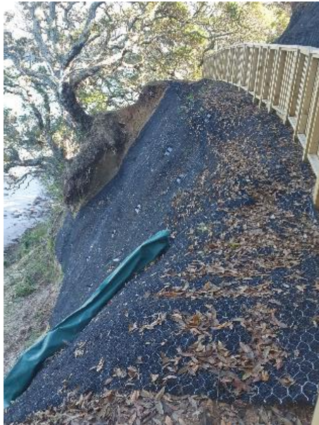
Photograph 6- View of slope looking west
