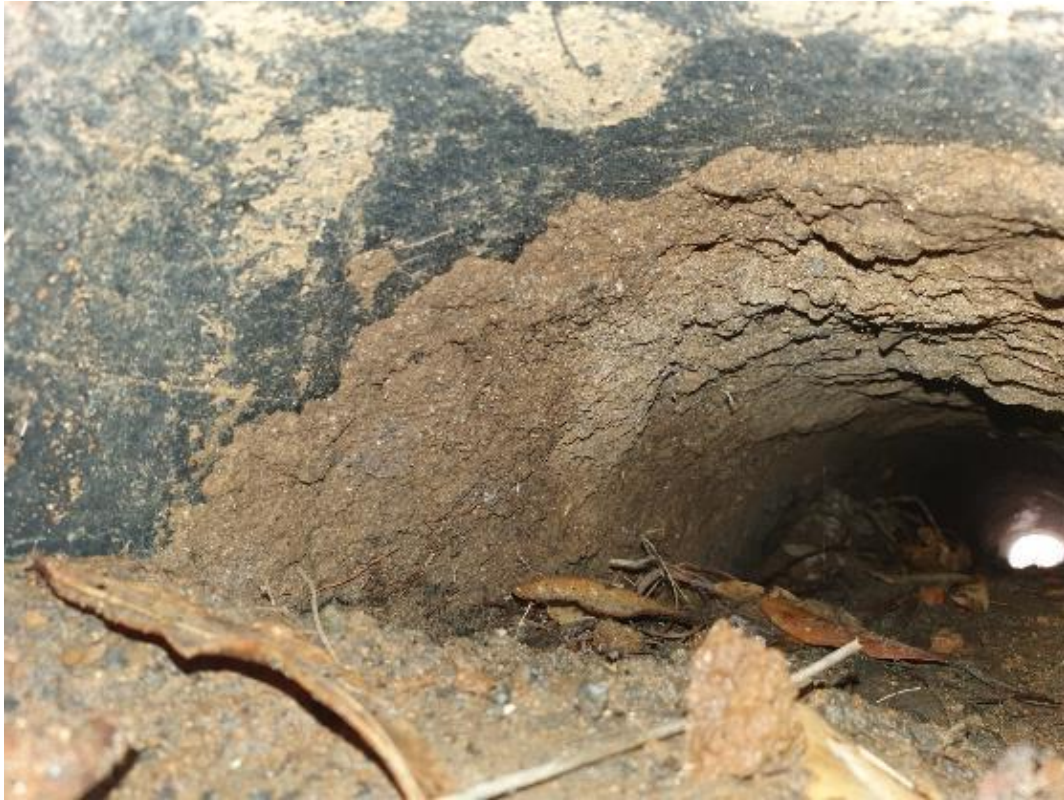
Photograph 5 - View inside Culvert 2 from track to edge of slope
