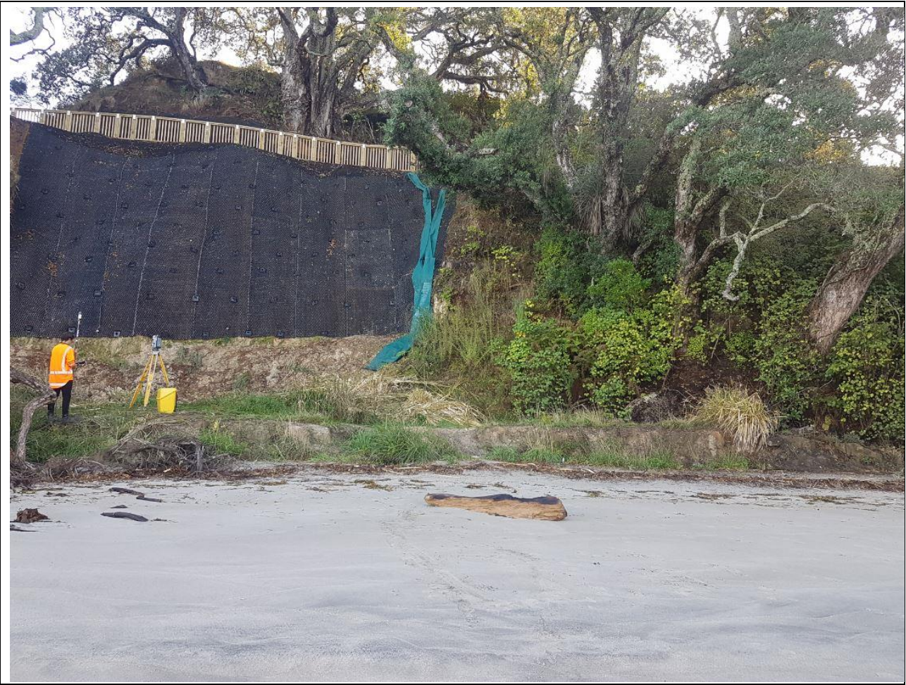
Photograph 17 – Survey team surveying the slope
