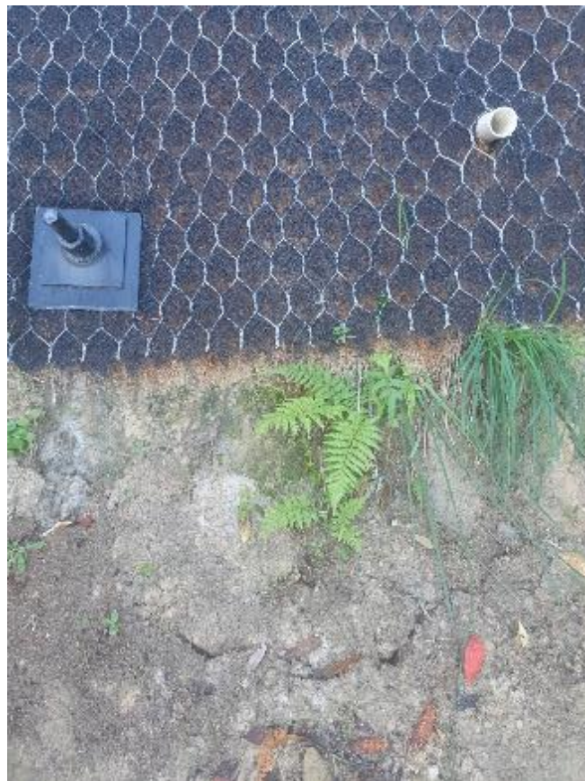
Photograph 10 - Horizontal drain O8 with slight cracking in material below
