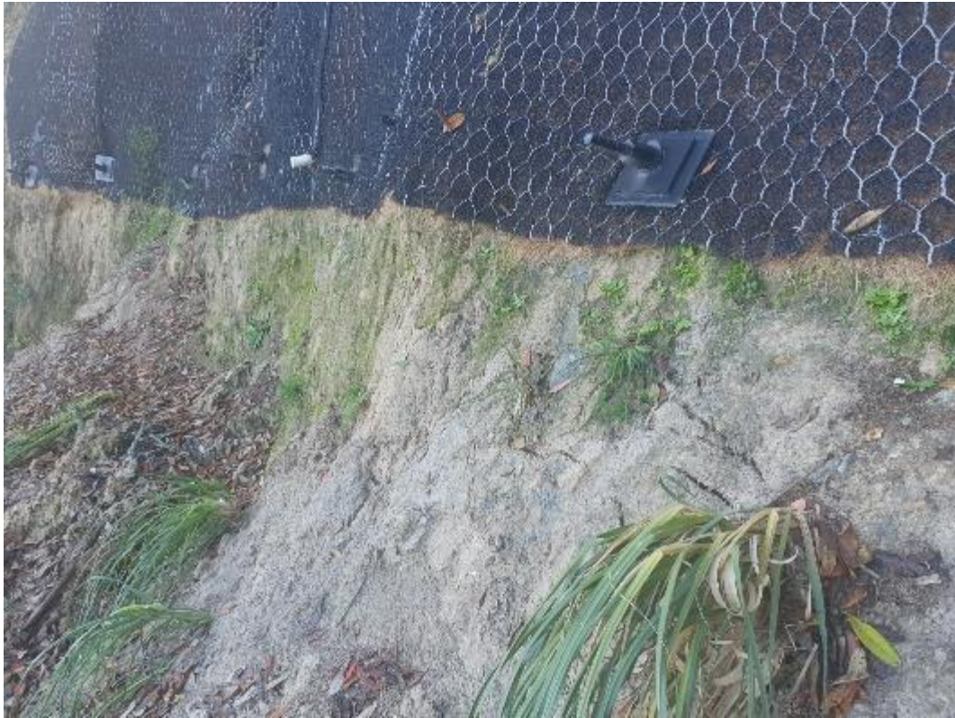
Photograph 11 - Looking east from horizontal drain 08 to horizontal drain 07
