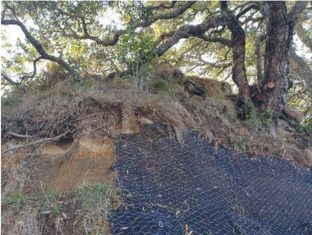
Photograph 15 - looking up to the slope above the top of the track
