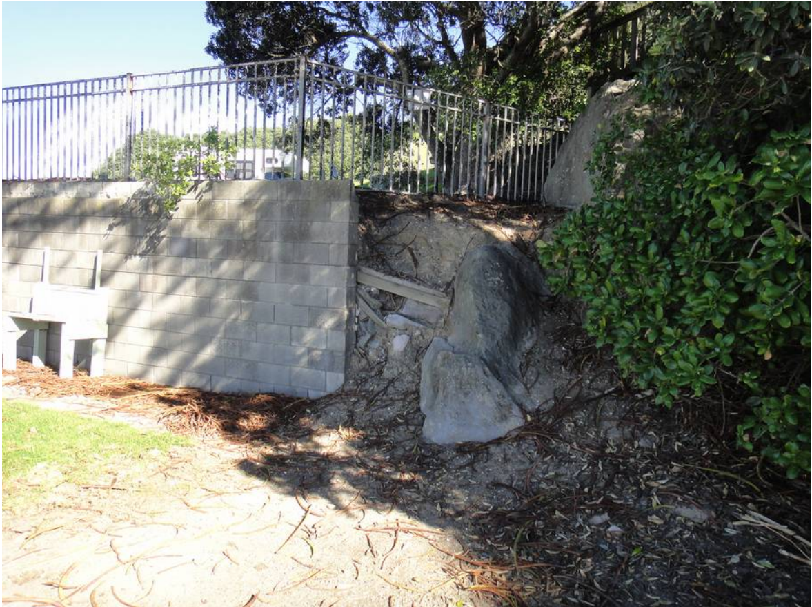
Photo 11; Retaining wall at northern end of campground.
