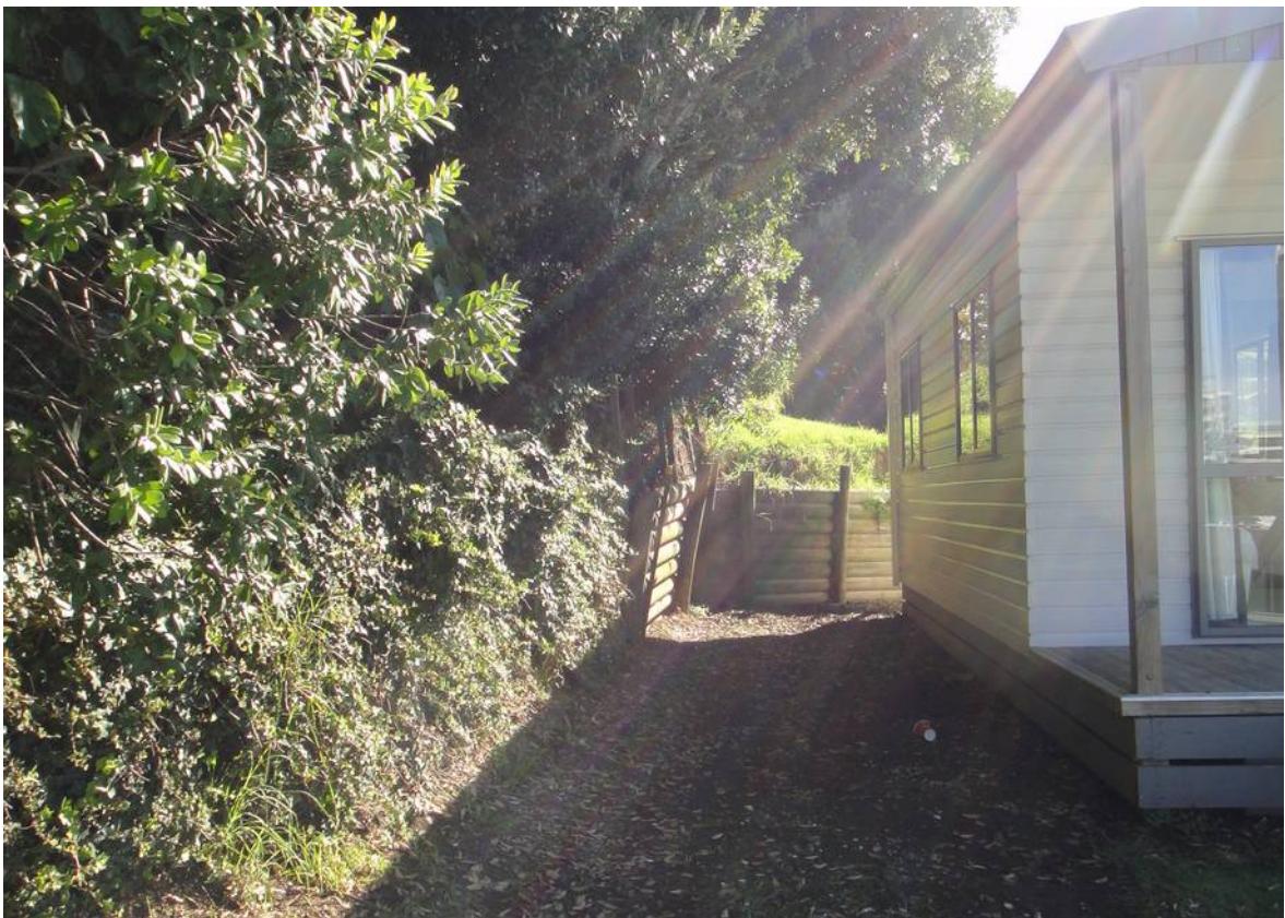
Photo 12; Retaining wall behind highest cabin.
