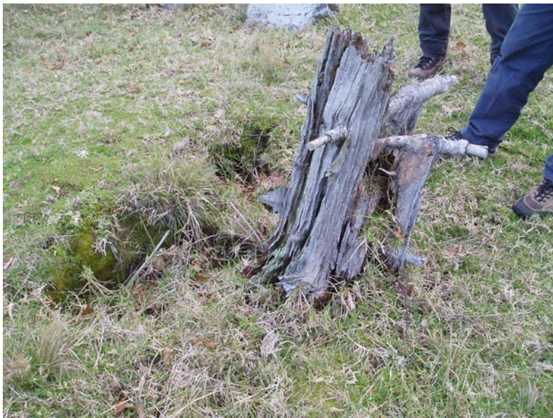
Photograph 3. Localised subsidence due to decaying root systems.
