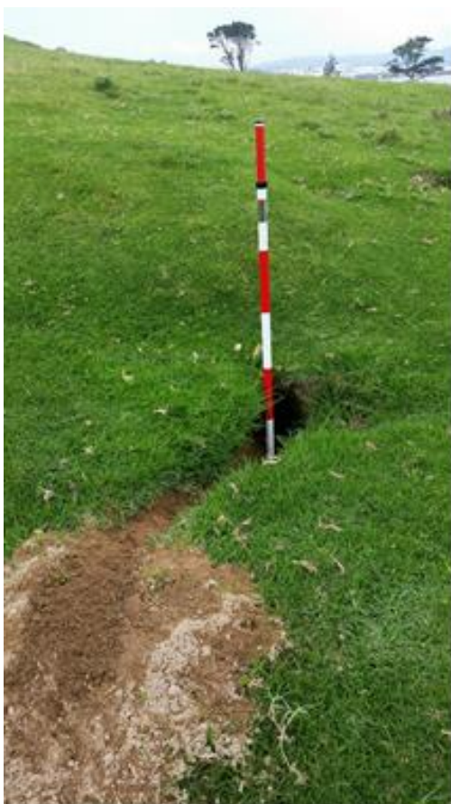
Figure 5: Example of damage caused by rabbit burrowing.
