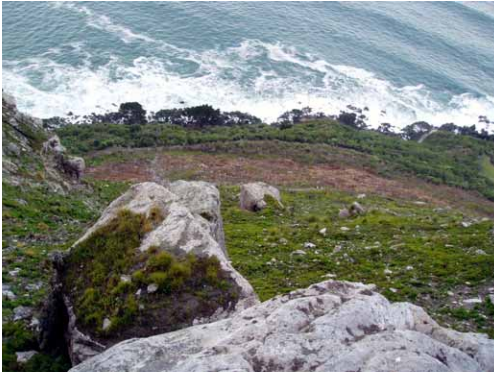
Photograph No 22; Unstable column at 3d.
