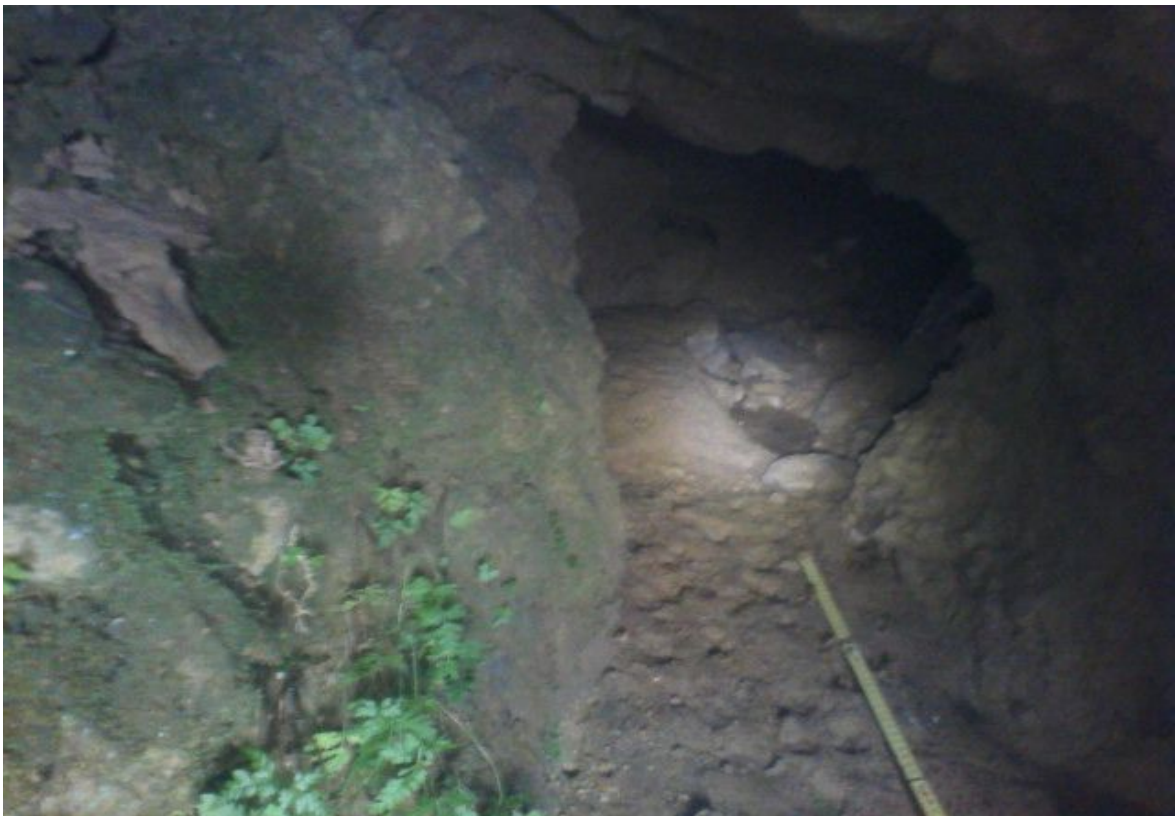
Photo 4; Looking further in the 'tunnel' appears to continue to the right. A small pool of water can be seen on the floor.
