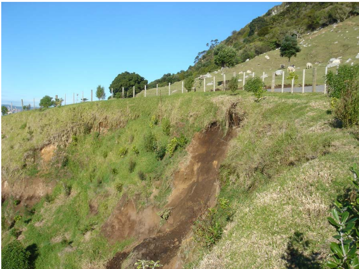
Photograph 1; Minor shallow slipping continues (slip 34)
