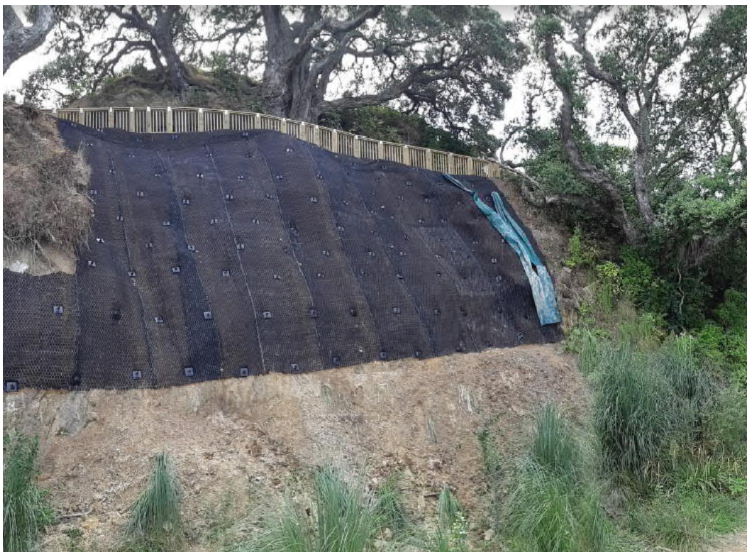
Figure 1: Soil Nails on southern side of Mauao.
