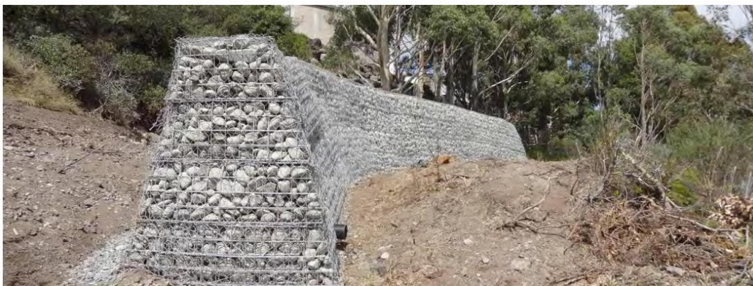
Figure 3: Typical mechanically stabilised earthbund rockfall barrier (source MBIE)
