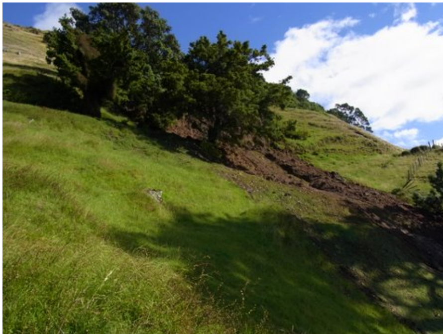
Shallow surface failure
