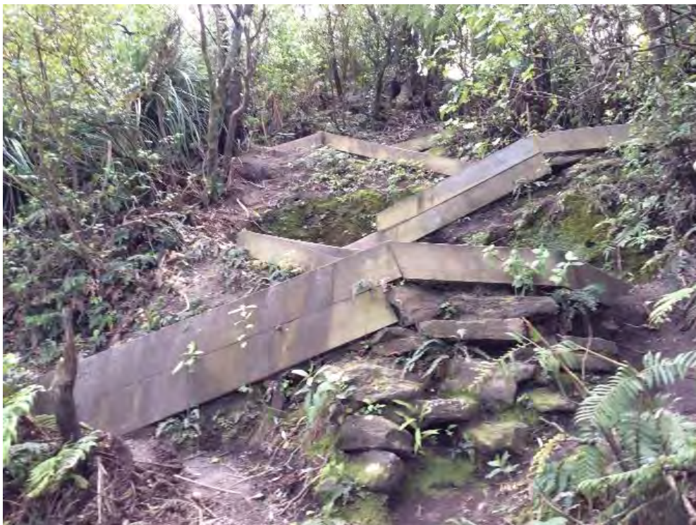
Figure 59: Connecting the Motu Kauri track to the Waikorire track there is a series of winding, steep steps through bush. It is recommended that the steps are maintained by removing any excess material and levelling the tread. Ensure that all wood is structurally sound and not rotting, if so, replace.
