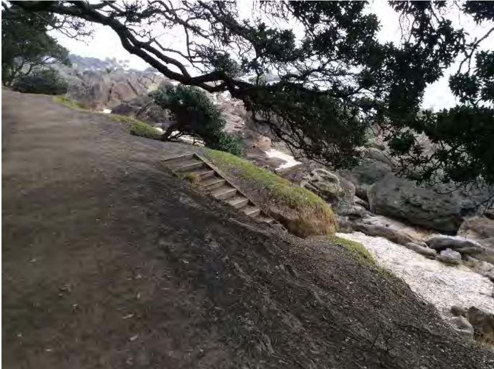
Figure 5: Formal access to Shelly beach lying beneath the base track. These steps are located in high visibility areas for safe access. Excess material can accumulate on the tread of the steps so it is recommended that this is maintained.
