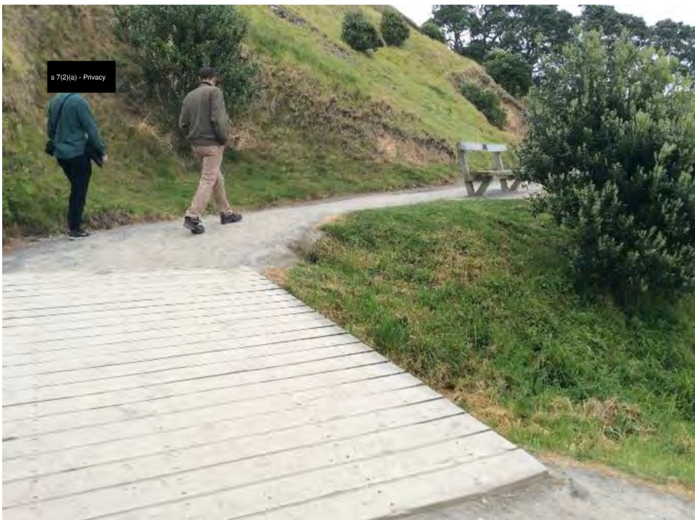
Figure 34: Small bridge that traverses a gully is one of the few built elements on Mauao's tracks excluding furniture.
