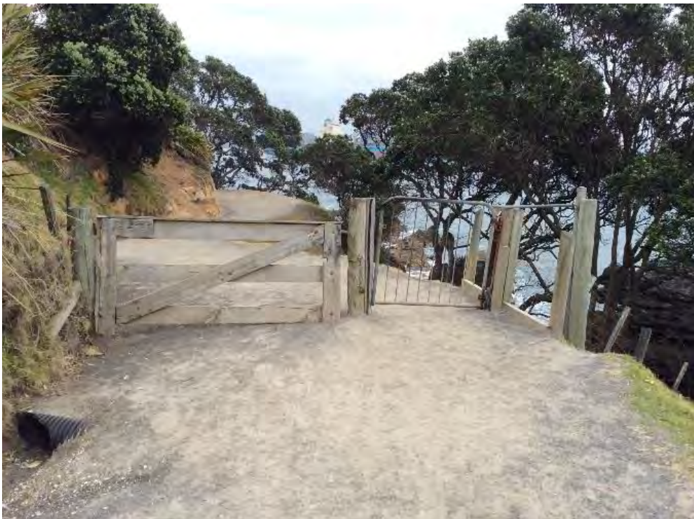
Figure 16: Vehicular and pedestrian gate are located along Mauao's base track. These gates are installed to keep the sheep stock contained. The vehicular gate is only unlocked in emergency cases.
