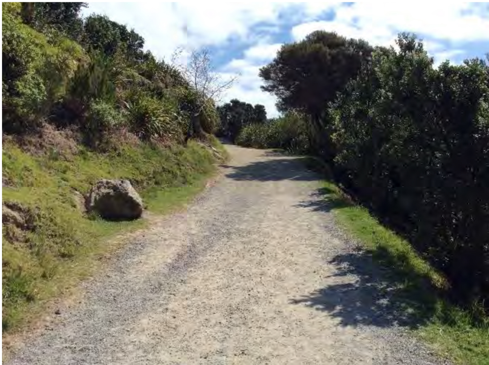
Figure 78: Access leading up to the junction with the Waikorire track is a gentle grade with a wide track, however, from the stone steps up to the junction the ground material is a GAP 40 chip. This results in a much higher frequency of slipping as the larger chip moves more freely. It is recommended that this chip is replaced with the finer gravel.
