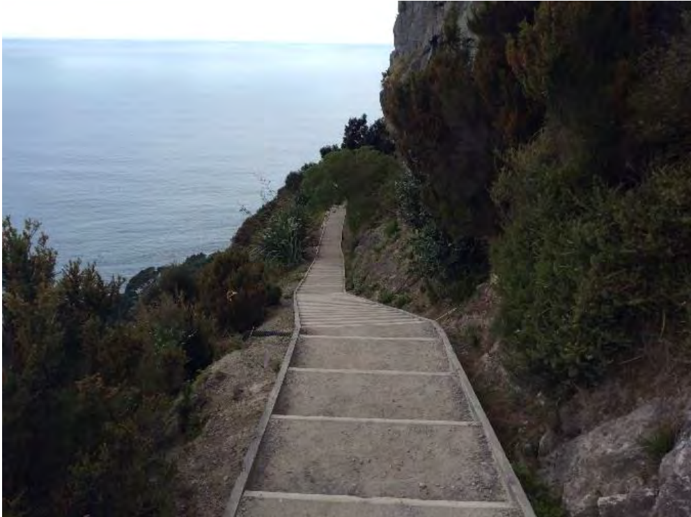
Figure 79: The upper section of the track consists of stairs that cascade down through a short section of bush and down an area on the cliff edge. The steps are well constructed with a good quality and well maintained ground material. Sightlines are clear for safety. Mountain flax is used as a soft border to define the steep cliff edge.
