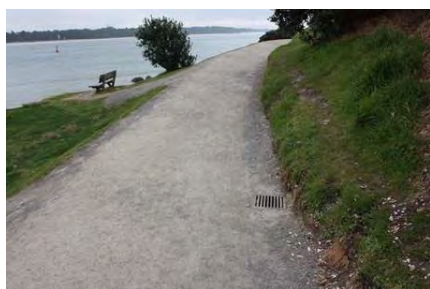
Figures 3, 4 and 5 Drainage holes on inward side of Base track and trial drainage cover
