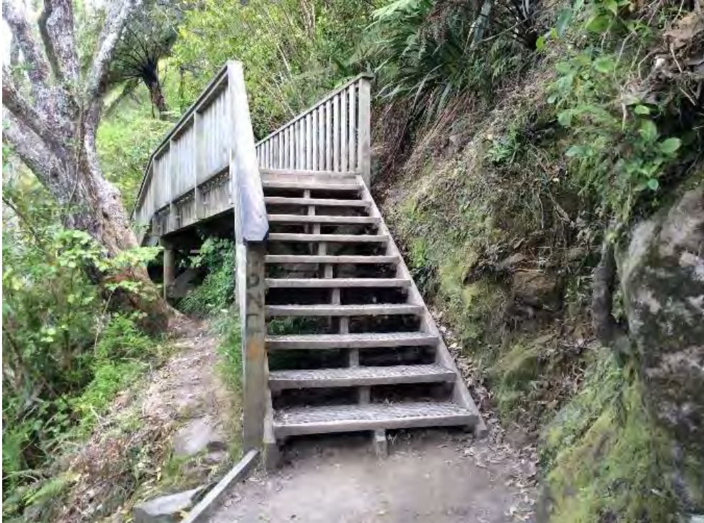
Figure 69: The bridge along the track is in good condition and is well constructed with good handrails and slip proofing. There is evidence of minor, old vandalism, however the design of the bridge is such that it provides very little areas for vandalism to occur or have a major effect.
