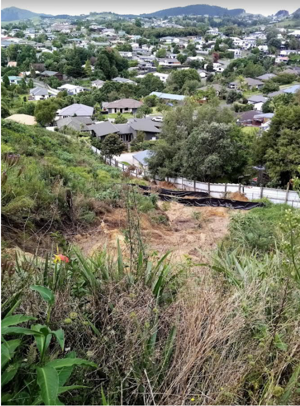
Figure 2: Path of debris flow
