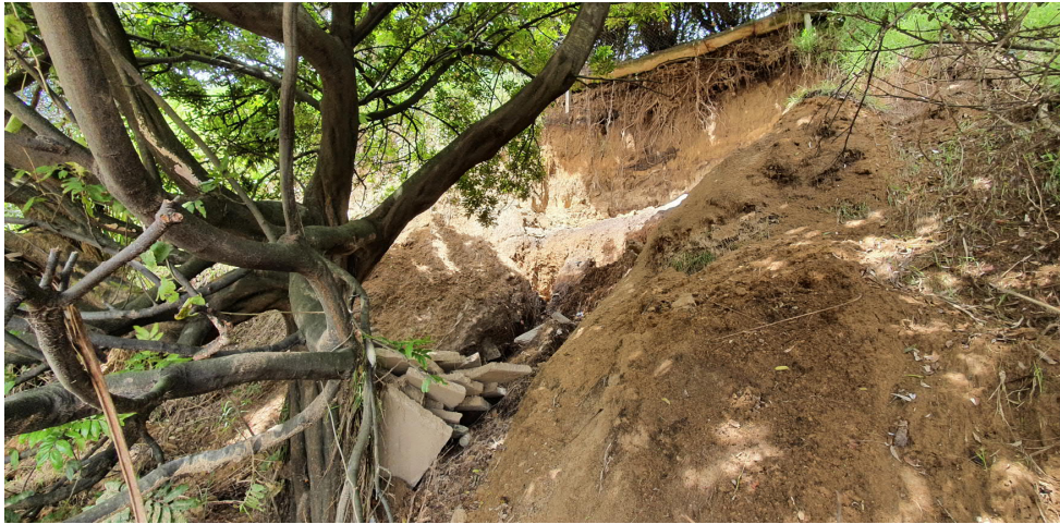
Figure 1: Slip failure with fill material below.
